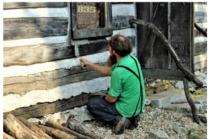
Vintage logs from a cabin in southern Missouri have replaced the rotted logs, and the area was rechinked by Miller's crew in late July.
