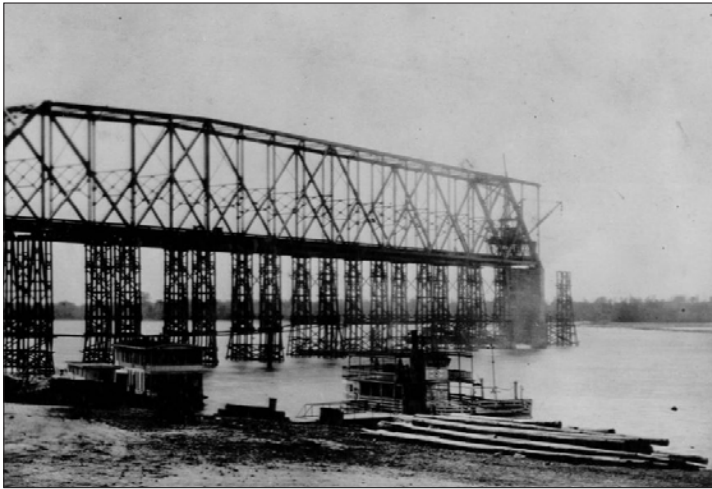
Erecting the main span of the continuous truss of the Memorial Bridge.
