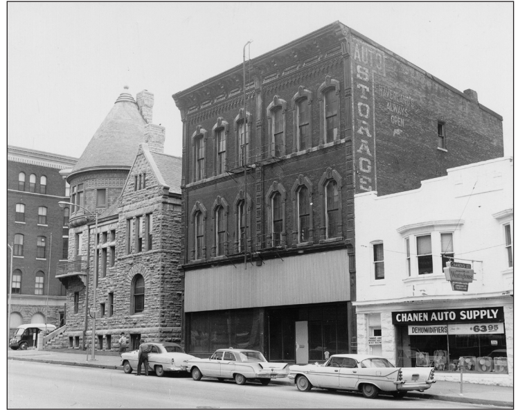
The Powers & Finlay building (center) was razed in 1965, and excavation for the Museum's new addition has just uncovered much of the demolition debris which was used to fill in the foundation.
